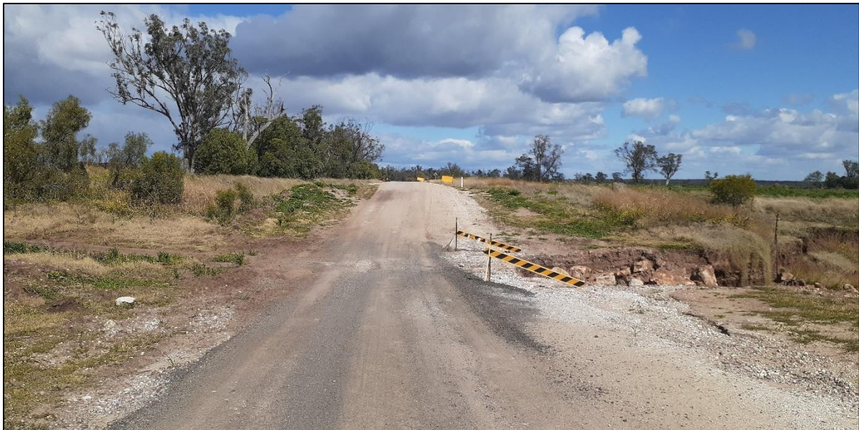
Figure 7: Example of road culvert damage along Melburra Road resulting in narrowing of road pavement
