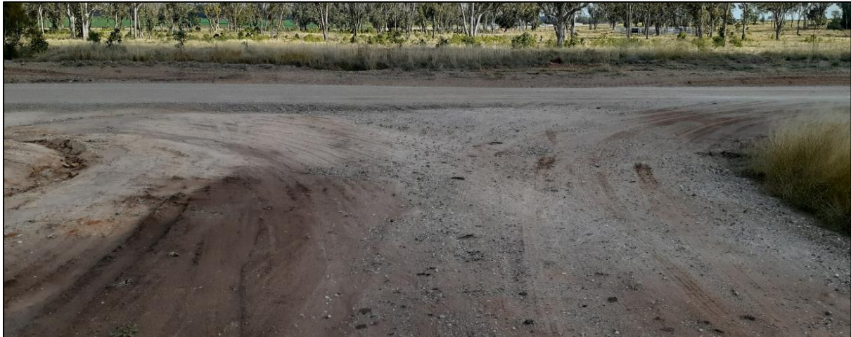
Figure 10: Melburra Road intersection from the quarry site showing limited gravel on left hand turn area.
